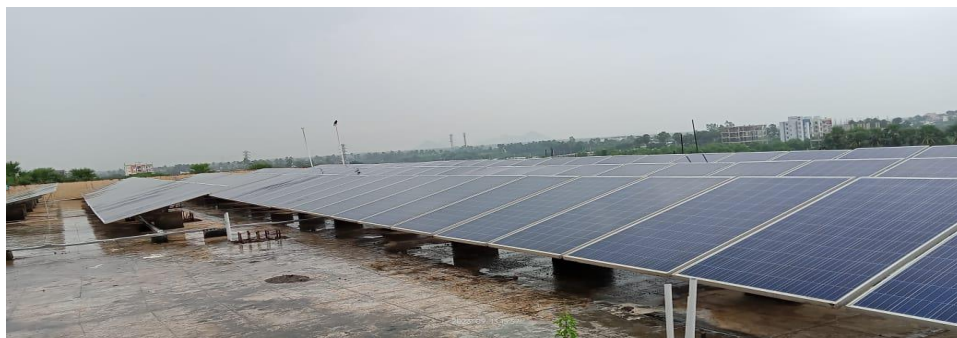
80 Solar Panels installed on the roof of Block 1
